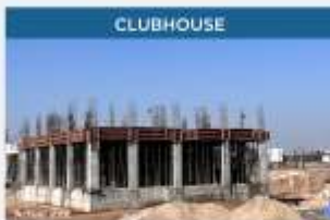
Clubhouse construction in progress
